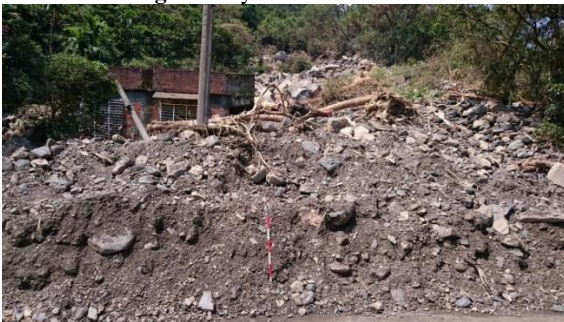
Fig. 2 Debris flow deposition in downstream reach in Ping-Guang Creek watershed (2015/08/13)
