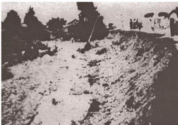
Fig. 12 Dike breach
