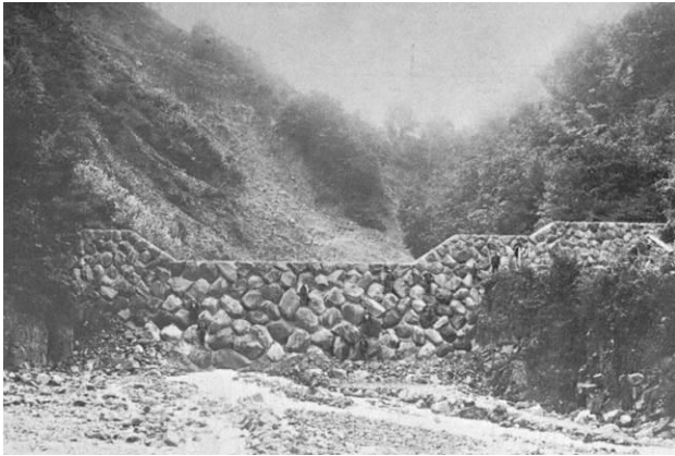
Fig. 15 No. 28 Sabo Dam of the Yomase River (constructed in 1924)
