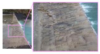
Fig. 8 Deterioration at the crest of the dam
