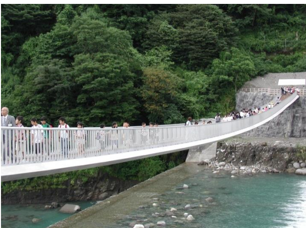
Fig. 16 Hongu Sabo dam maintenance bridge
