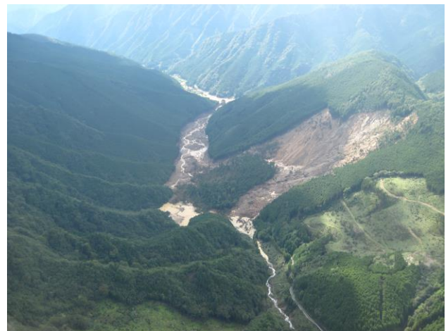
Fig. 3 Damage situation of the Iya area
