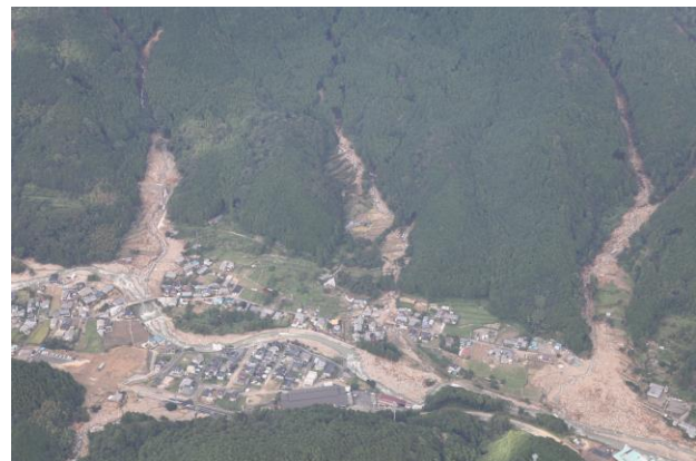
Fig. 4 Damage situation of the Nachikatsu-ura town
