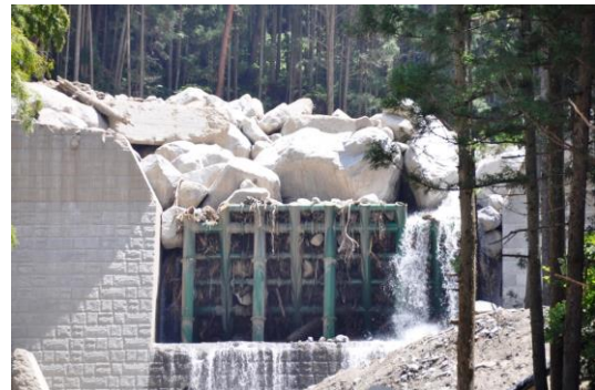
Photo 1 Steel open Sabo dam
