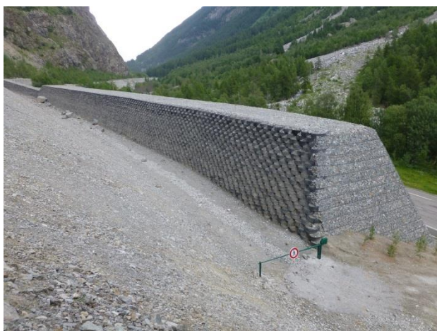
Fig. 1 Example of a 7m-tall reinforced embankment protecting a road (S. Lambert)
