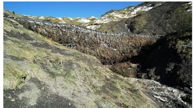
Figure 10: 11 debris flow protection barriers, successfully filled in Hasliberg in 2011.
