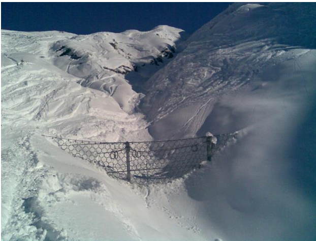
Figure 4: Same net than in figure 3, partially snowed in during winter. The snow load has to be taken into account when designing the barrier.
