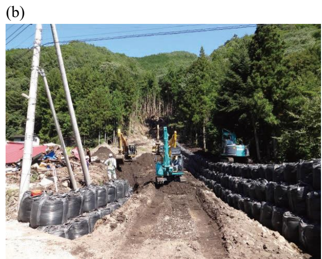
Fig. 15 Emergency construction (a) Right after the disaster (b) A temporary diversion channel is constructed with large sandbags
