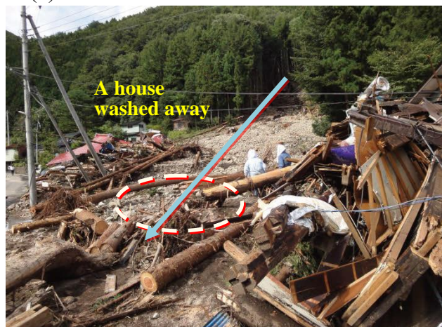
Fig. 6 Damage in Takimukaisawa, Serizawa District (a) Sediment and driftwood run off (b) A damaged house (two people injured and three houses completely destroyed)
