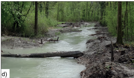
Figure 1d: Flood mitigation and restoration project Aare River: right bank natural secondary channel
