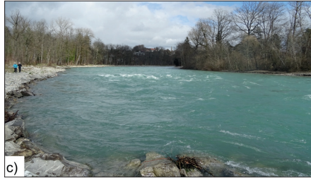
Figure 1c: Flood mitigation and restoration project Aare River: right bank enhanced state
