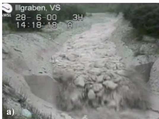
Fig. 11 a) overtopping of a check dam by a debris flow (WSL, 2000), b) correlation of stress due to fluid shear and slope angle, comparison of 2 models, marked area is decisive for the Lammbach check dams.
