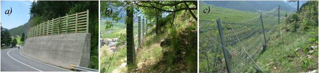
Fig. 2 Falling rock protection barriers within the Autonomous Province of Bolzano: a) and b) low capacity systems, c) high capacity systems
