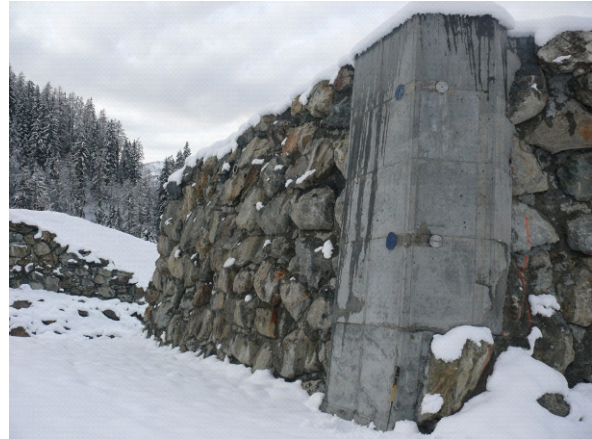
Fig. 9 Breaking mound (7,5 m high) with pressure and velocity sensors
