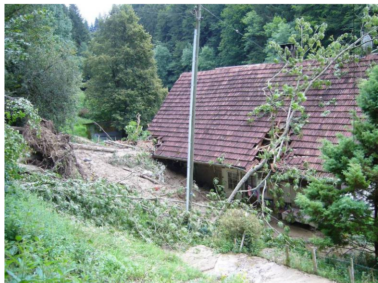
Fig. 9 The debris flow of 8 August 2008 in Köniz. Many trees were uprooted and probably acted as point-loads against the house
