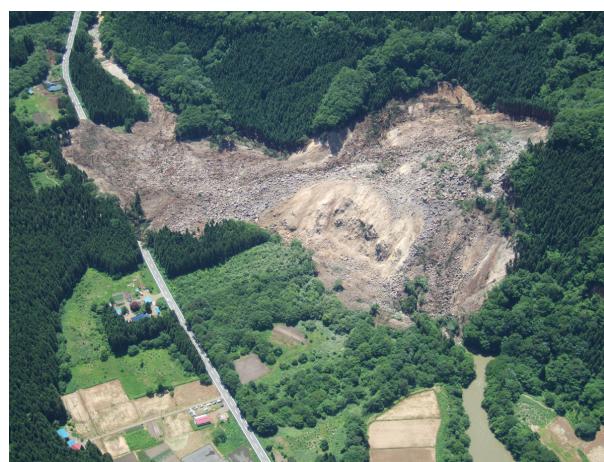
Fig.4 Slope failure and landslide dam at Azabu, Ichihasama River
