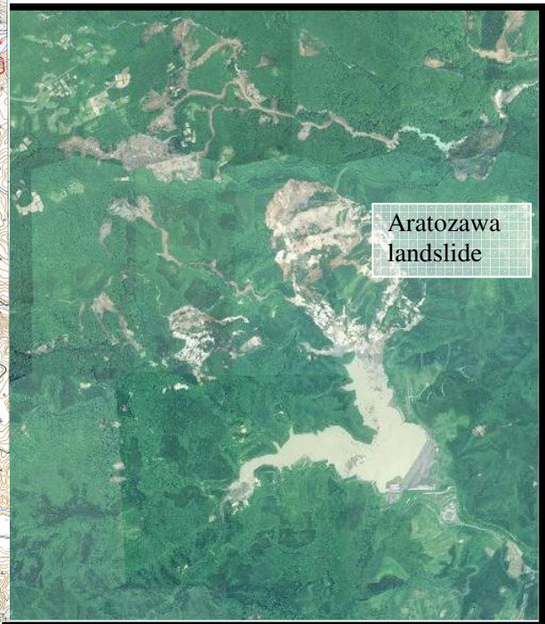
Fig.6 Aerial photograph after the earthquake taken by Asia Air Survey Co. Ltd
