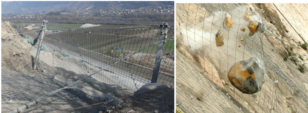
Figs. 1 Catchment area of attenuating structure (left) and guided boulder along rock face (right)
