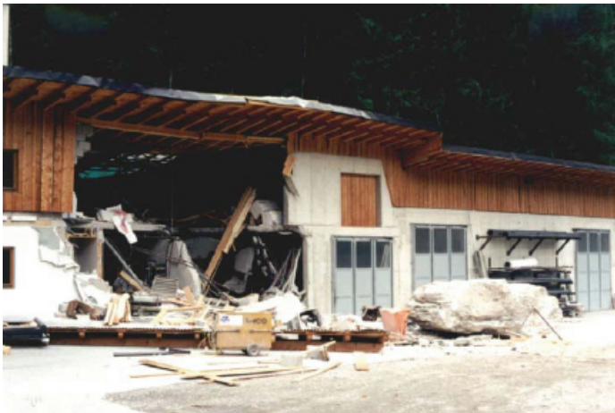
Fig. 1: Rock fall event in 1998 destroying a building in Zillertal, Tyrol, Austria
