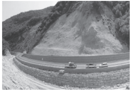
Fig. 12: Intervento sulla frana in detrito Fig. 12: Consolidation of roto-translational earth slide
