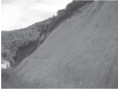
Fig. 11: Consolidamento con soil nailing Fig. 11: Soil nailing
