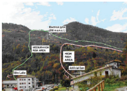
Fig. 14. Front view of Idro landslide with the limits of high risk area.
