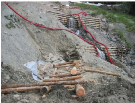
Fig. 10. Wooden crossbeams view during the construction.
