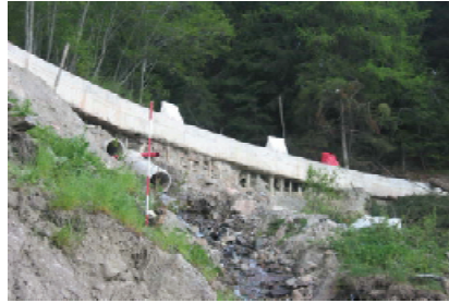
Fig. 4. Uncovered micropiles.
