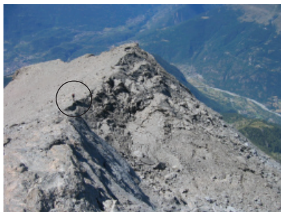
Fig.8: Western Rocciamelone crest. Since 2006, rock slope deformation became apparent, arising concern about a possible collapse. The person in the circle is for scale. Photo by P. Intropido.
