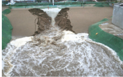
Photo 8. Collapse of a landslide dam (60 m in height) by erosion.
