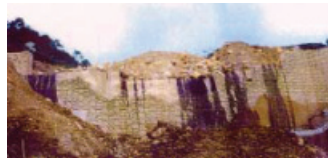
Fig.1: Debris flow disaster
