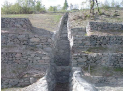
Fig. 13: view of the drainage channel
