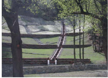
Fig. 14: view of alternative drainage works
