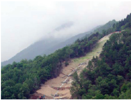
Fig. 7: Upper reach of the conoid, Biodegradable mats and hydro seeding
