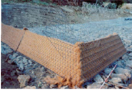
Fig. 16: Rovarey, deflecting wall at the beginning of construction
