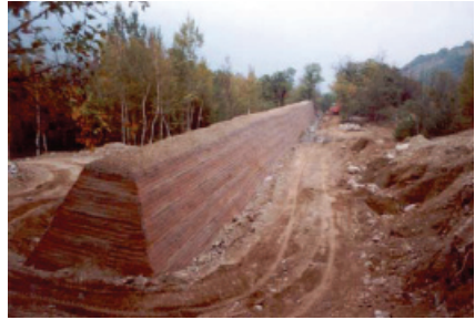
Fig. 17: Rovarey, deflecting wall at end of construction
