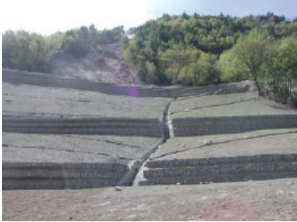
Fig. 9: overview of gabion drainage works
