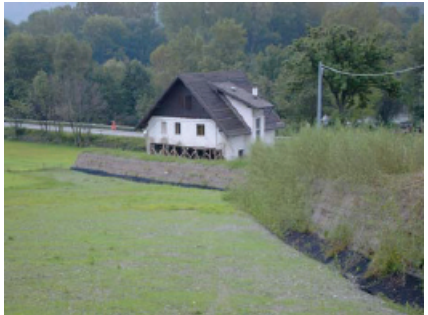
Fig. 19: Nus, deflecting wall at downstream end
