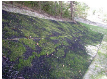
Fig. 8: Upper reach of the conoid, Turf reinforcement mats and hydro seeding
