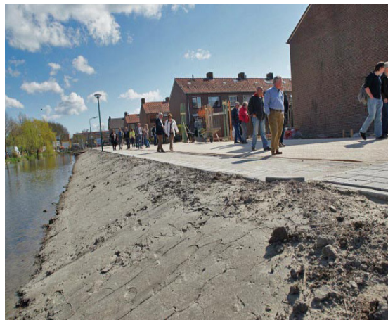
Elevated street after reconstruction. Credits: G. Kleinveld
