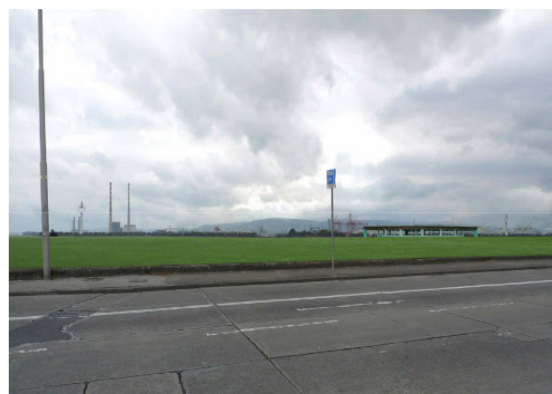
View 2. Top: existing view of Clontarf promenade along Fortview Avenue. Bottom: proposed flood defences and view of Clontarf promenade along Fortview Avenue. Credits: Dublin City Council
