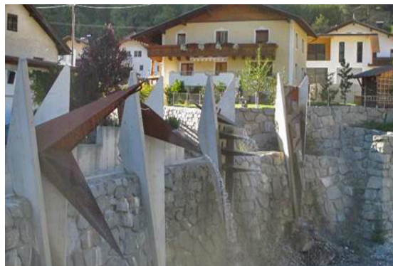
Fountains in the flood retention basin. Credits: S. Fuchs
