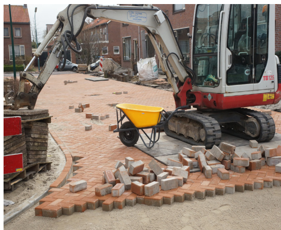
Construction of street elevation. Credits: G. Kleinveld
