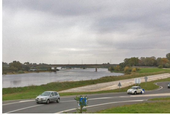
Fuse wire of the Bouillie spillway. Credits: M. Galepois
