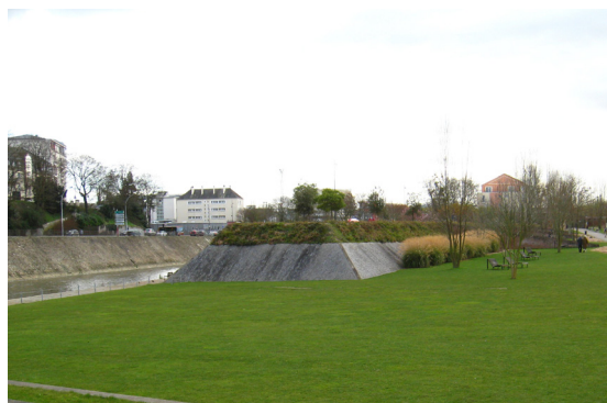
Le Mans, France: Île aux Planches as an example for flood mitigation with multiple use. Credits: S. Fuchs
