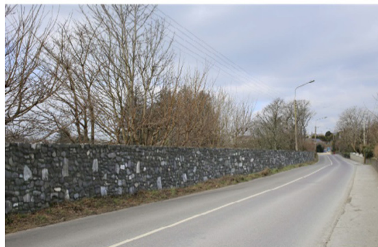
Top: Existing view entering Skibbereen. Bottom: view entering Skibbereen on completion of current structural flood relief works. Credits: Office of Public Works
