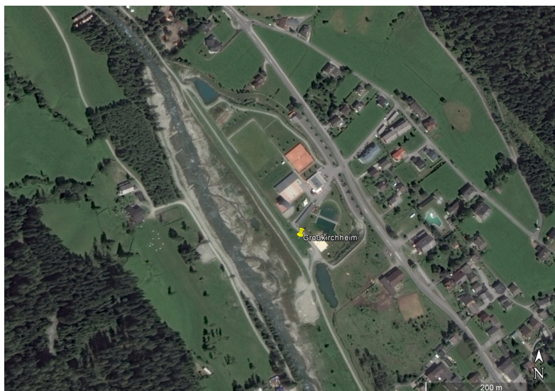
Großkirchheim flood protection. Credits: Google Earth
