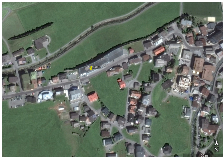
Galtür avalanche dam. Credits: Google Earth
