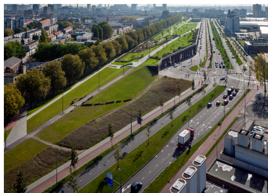
Rooftop park after completion. Credits: S. Brakkee
