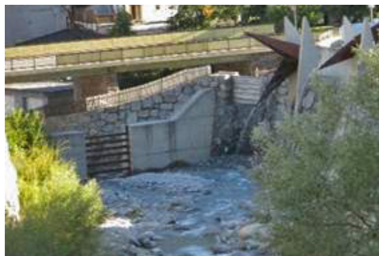
Pfunds flood retention basin. Credits: S. Fuchs
