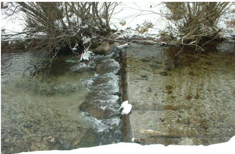
Foto 6: Holzschwelle vor Umbau (Untersuchungsstelle 3) Picture 6: wooden sill before reconstruction started (investigation area 3)
