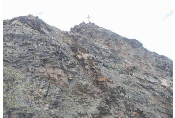
Rockfall scar. Photo: V. Mair
