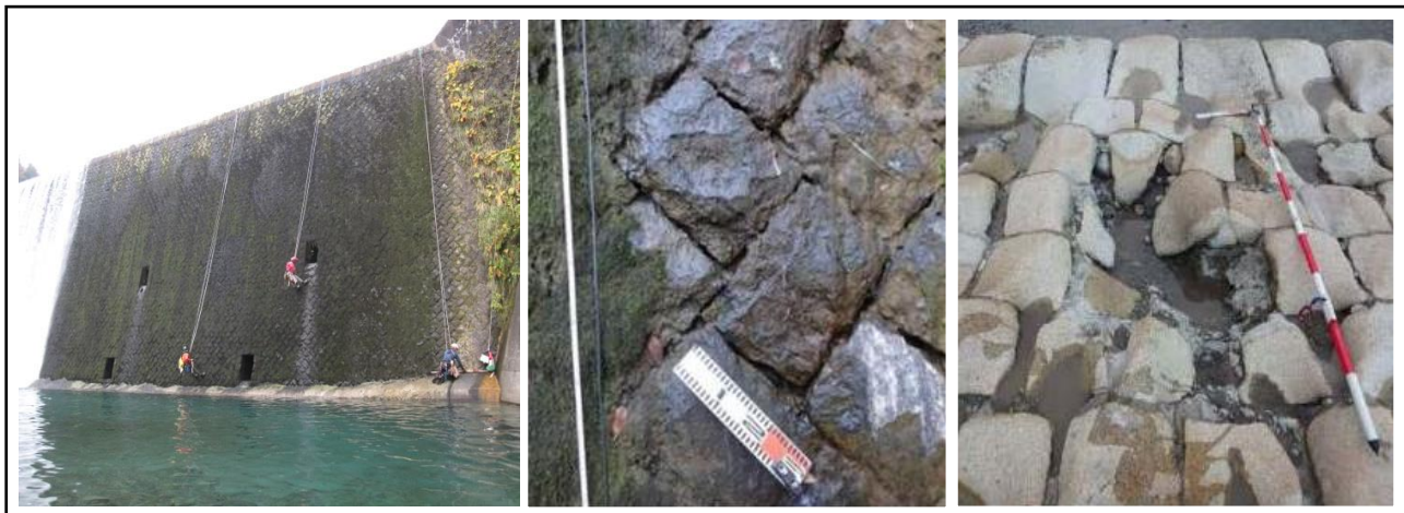
Fig. 10 Example images of detailed visual inspections of sabo facilities
