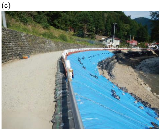
Fig. 14 Removing obstacles from the road (a) Removing sediment and driftwood (b) Damaged areas are temporarily repaired with large sandbags (c) Road temporarily restored
