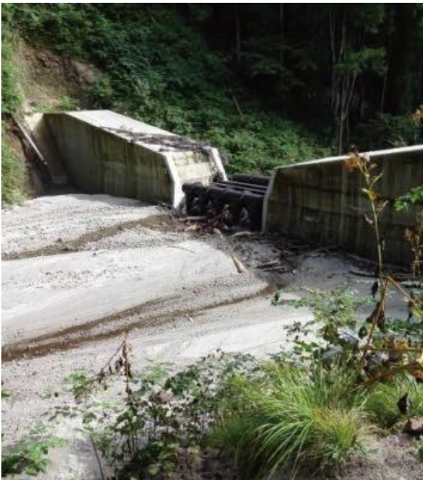
Fig. 11 Effect of an erosion control facility (Tamozaawa Erosion Control Dam 1)
