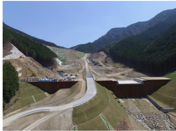
Fig. 5 Disaster prevention works of the Iya area
