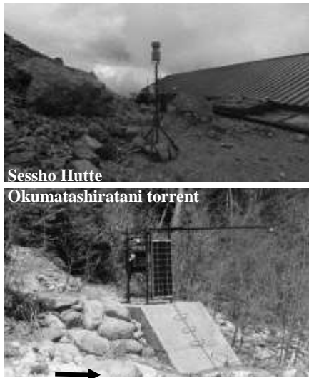
Fig.3 Installation of rainfall and water level gauges
