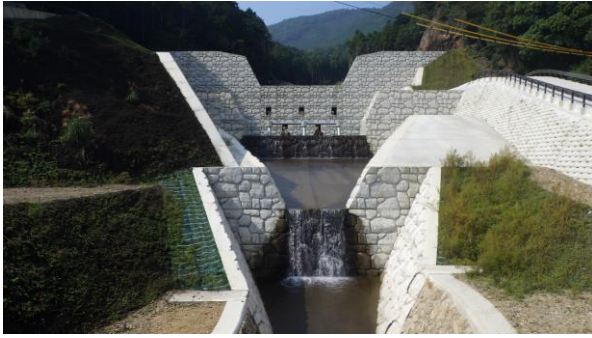
Fig. 7 Disaster prevention works of the Nachi-River basin
