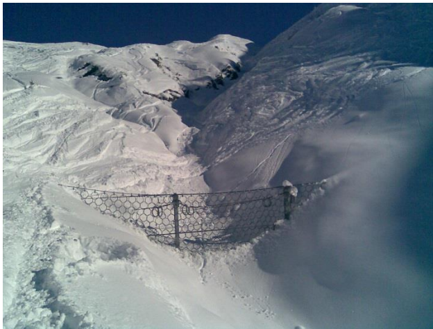
Figure 4: Same net than in figure 3, partially snowed in during winter. The snow load has to be taken into account when designing the barrier.
