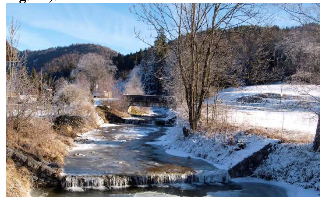
Fig. 12 Bridge at Entfelderstrasse
