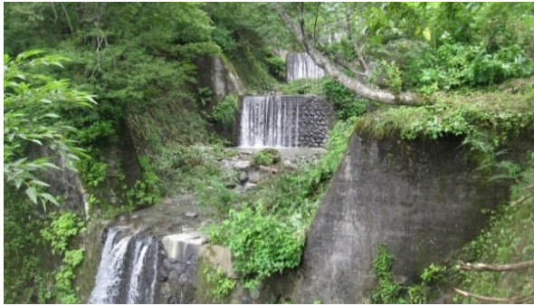
Fig. 6 Dorodani Sabo Dams (under construction)
