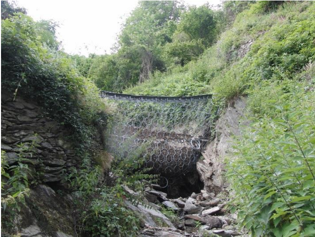
Figure 8: Partially filled debris flow barrier above the German Railway close to Koblenz.
