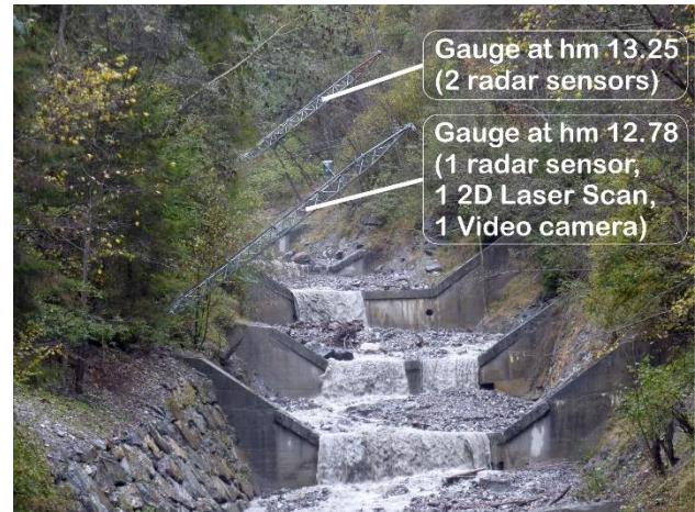
Fig. 2 Monitoring site “Grins” in the middle reach of Lattenbach, consisting of two single steel supports made of Garaventa elements with mounted sensors.
