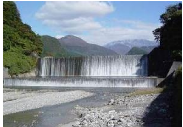
Fig. 3 Hongu Sabo Dam
