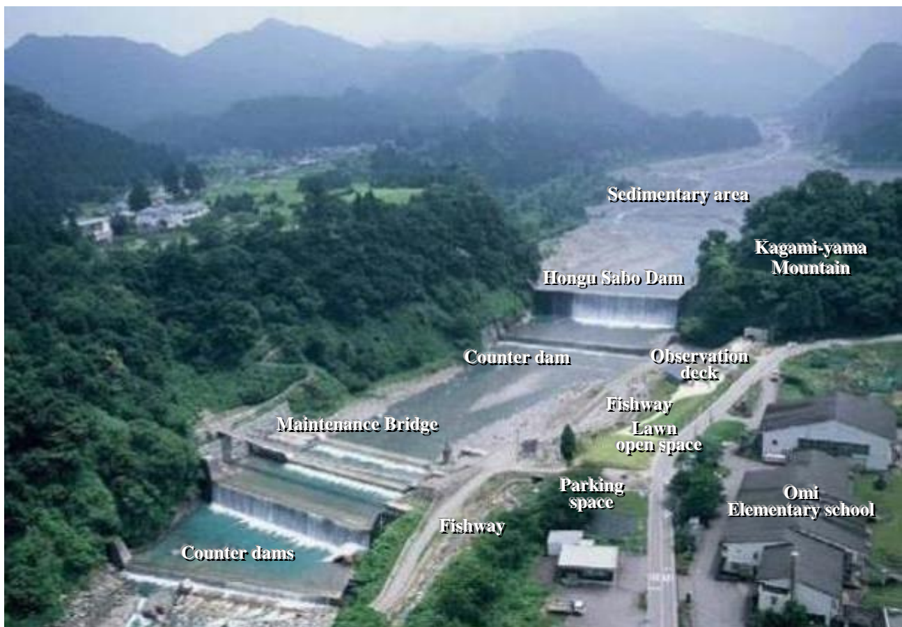
Fig. 19 Environmental improvement around Hongu Sabo Dam
