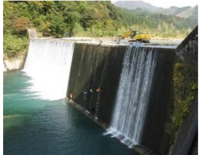
Fig. 10 Detailed visual inspection
