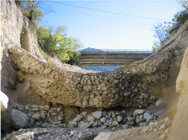
Figure 1: Testing of debris flow retention system with ring net in the Illgraben channel, 2006. Retention volume approx. 1000 m 3
