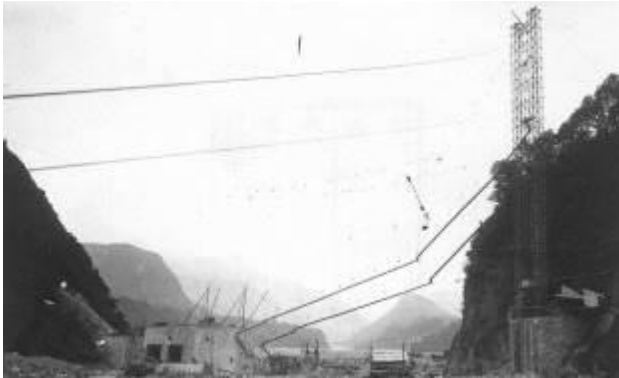
Fig. 4 Large tower cranes and chutes (1935)
