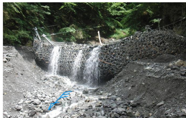
Photo 5 An example of capture of debris by the flexible debris flow barriers
