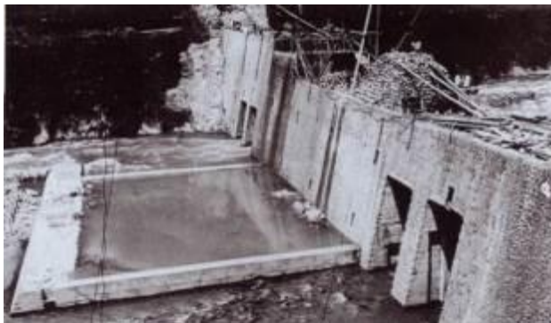
Fig. 5 Hongu Sabo Dam construction (1936)
