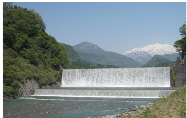
Fig. 5 Hongu Sabo dam (present day)
