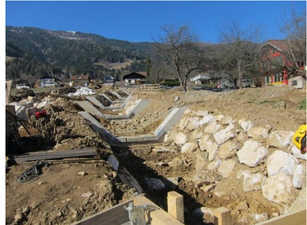
Fig. 10 Bedded rockfill and concrete sills along the lower reach
