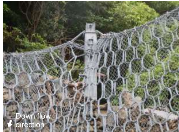
Fig. 19 Deformation of the ring net
