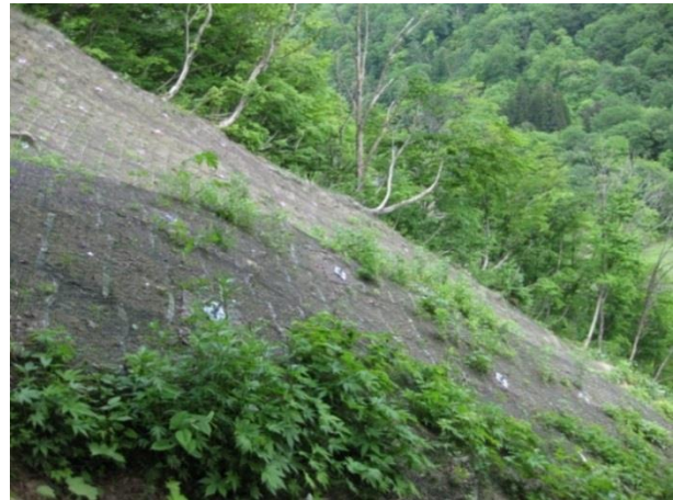
Photo 3 An example of slope stability works used by high tensile strength steel net
