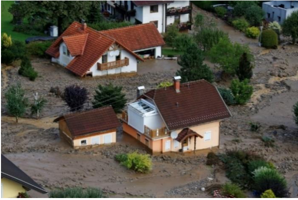
Fig. 6 Damaged buildings after the 2 nd debris flow on 4 th of September 2016
