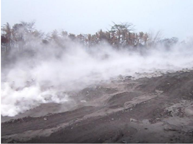
Fig. 7 Debris flow flowing in the guide channel under construction (December 30, 2010)
