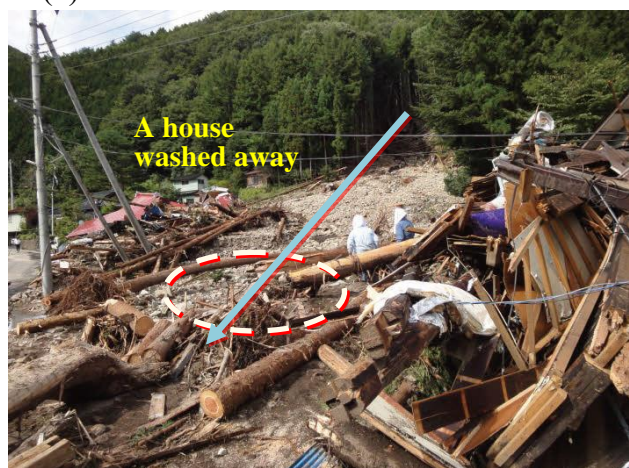
Fig. 6 Damage in Takimukaisawa, Serizawa District (a) Sediment and driftwood run off (b) A damaged house (two people injured and three houses completely destroyed)
