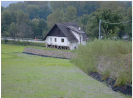
Fig. 19: Nus, deflecting wall at downstream end
