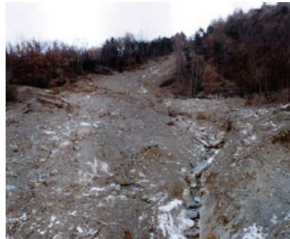
Fig. 2 : Oct. 2000 – Miseregne - View of main landslide from the uphill side down
