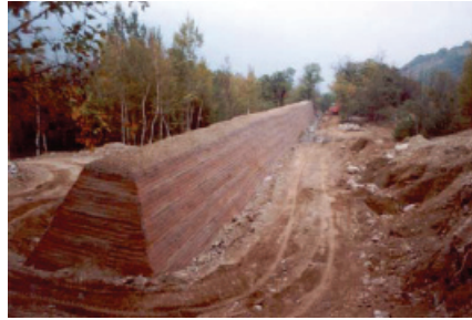
Fig. 17: Rovarey, deflecting wall at end of construction
