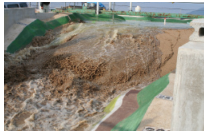
Photo 9. Collapse of a landslide dam (60 m in height) by rotational slide.
