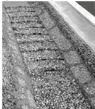
Fig8: Structured block ramp
