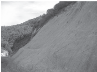
Fig. 11: Consolidamento con soil nailing Fig. 11: Soil nailing
