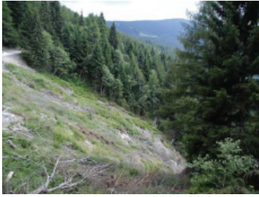
Fig. 3. General view of Vridel landslide.
