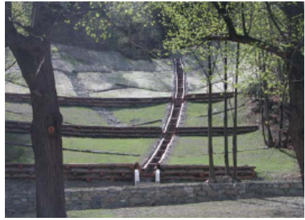
Fig. 14: view of alternative drainage works
