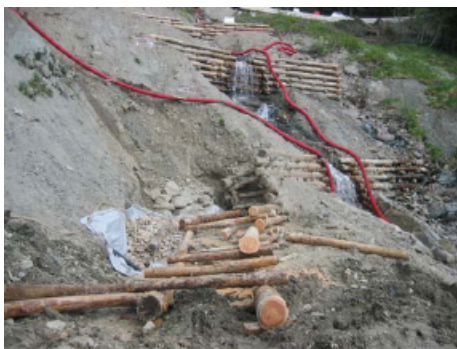
Fig. 10. Wooden crossbeams view during the construction.
