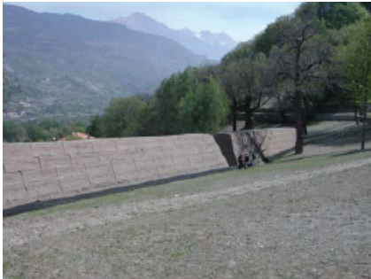
Fig. 18: Miseregne, openings to let the flow through without pressure build-up
