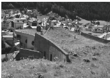
Abb. 13: Ebenhöf. Fig. 13: Roof terrace to integrate the building into the surface of the slope.
