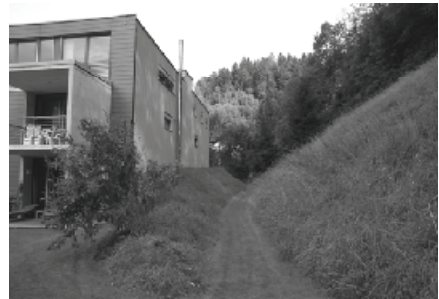
Abb. 10: Erddamm (Fallboden). Fig. 10: Earth-filled dam for energy dissipation of falling rocks.
