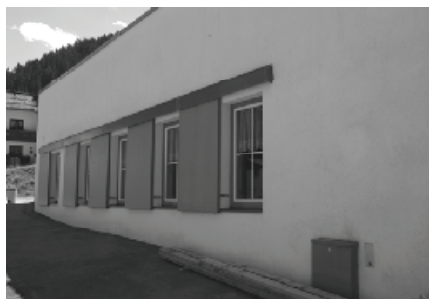
Abb. 14: Massive Fensterläden. Fig. 14: Window shutters to prevent intrusion of snow.
