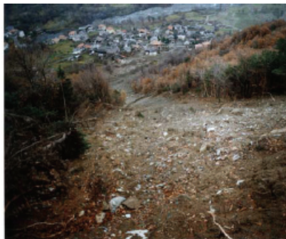
Fig. 3 : Oct. 2000 – Miseregne - View of main landslide from the uphill side down
