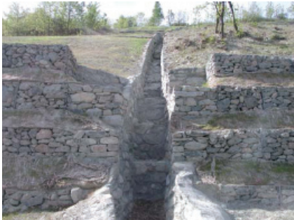
Fig. 13: view of the drainage channel
