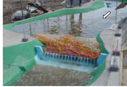
Photo 3. Upstream water level when a ground sill traps woody debris.
