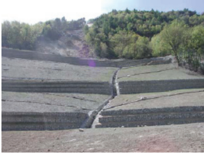
Fig. 9: overview of gabion drainage works
