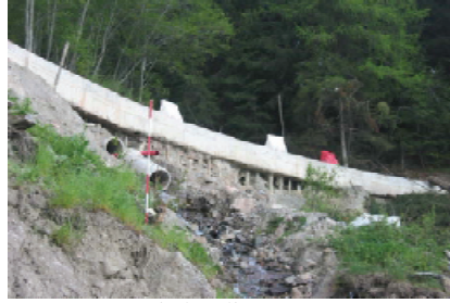
Fig. 4. Uncovered micropiles.
